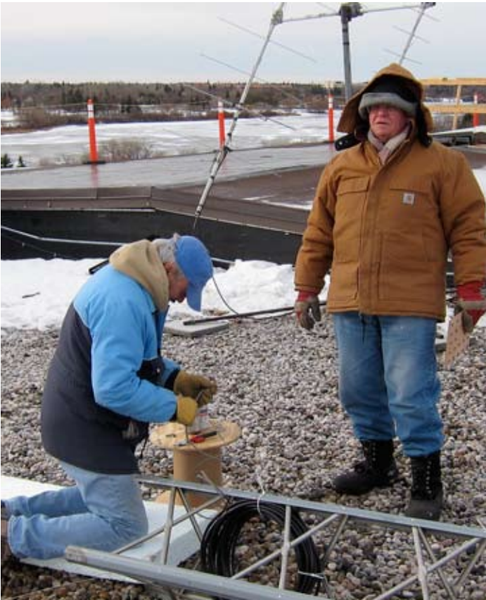
Malcolm working on connectors, Ron supervising
