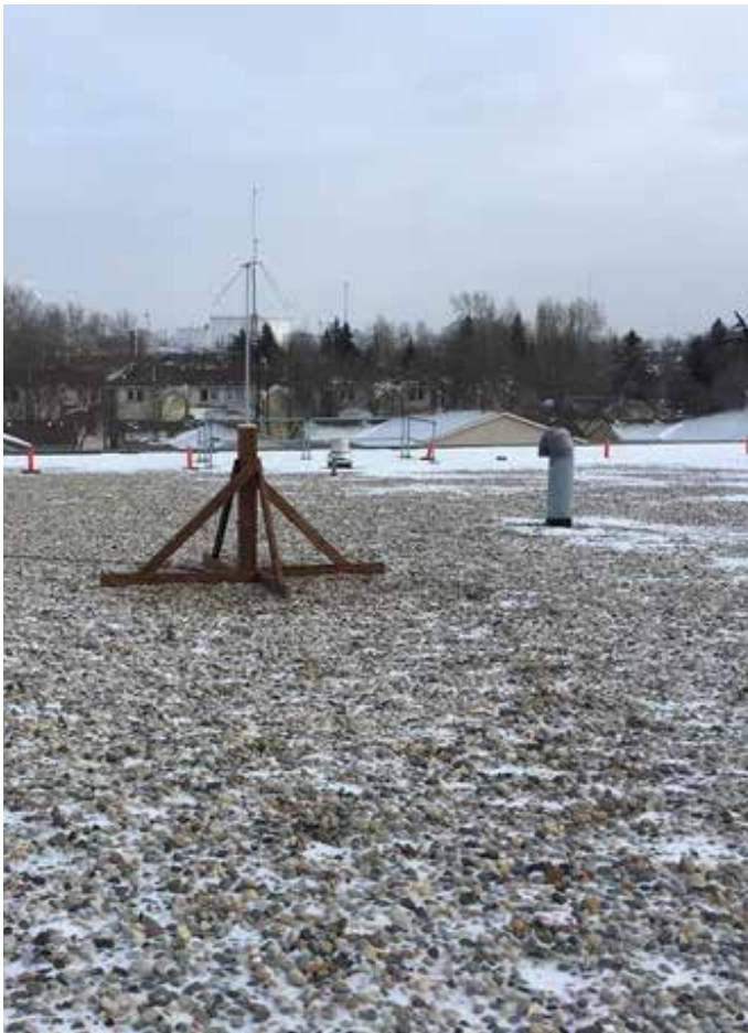
Photo showing temporary antenna base and 2 meter antenna
